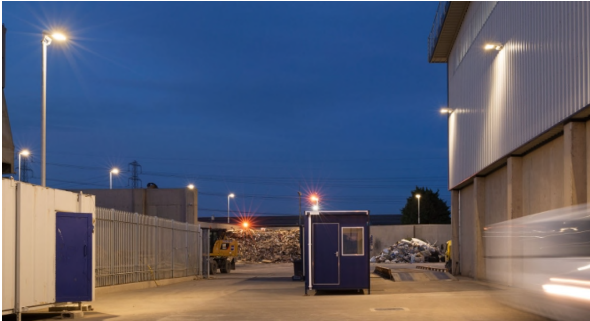
Figure 4.1: Example lighting in an industrial area
